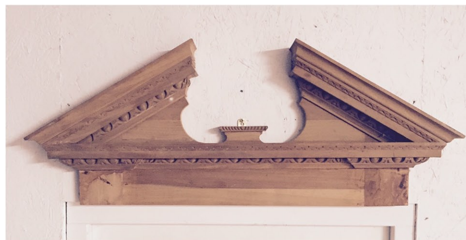
Broken Pediment over single door_Reference Picture
