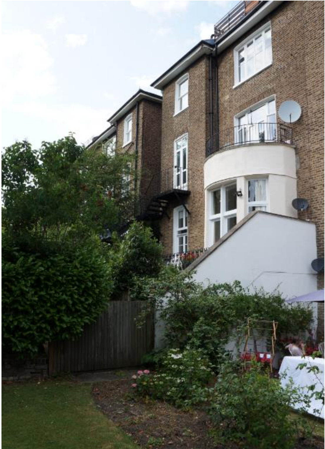
Photo 3: View to adjoining property no. 73
