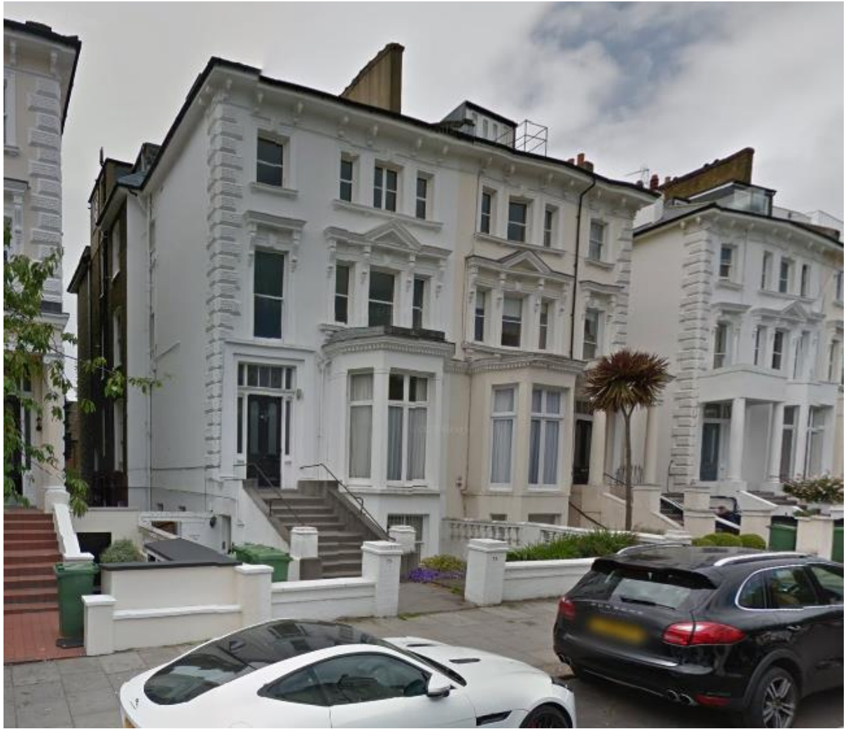
Photo 4: View showing side elevation and existing side dormer from street
