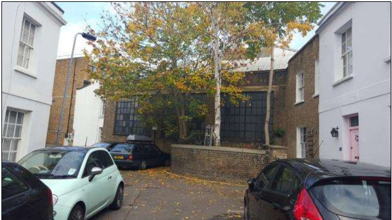
Figure 4: The southern elevation of B1.
