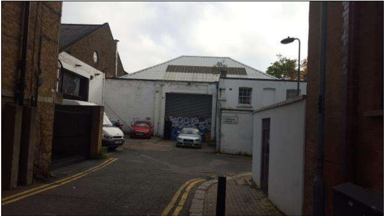
Figure 1: Looking east at B1 from the road.
