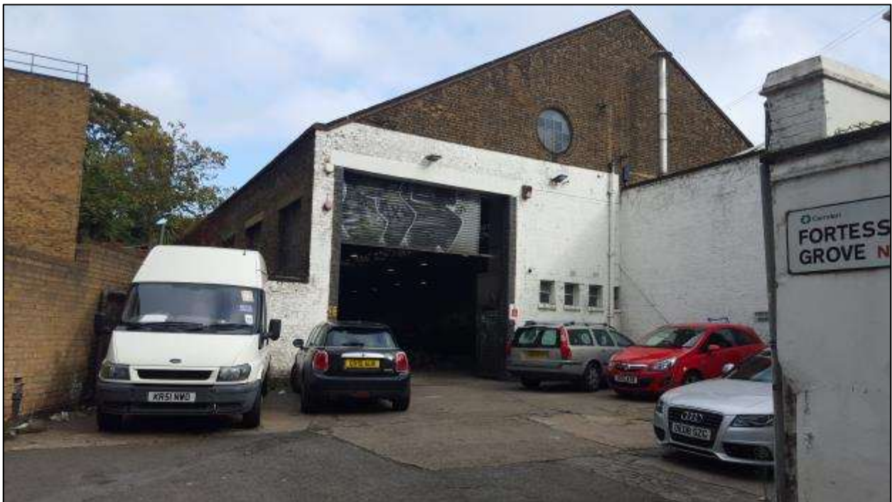
Figure 2: Looking north-west at B1.
