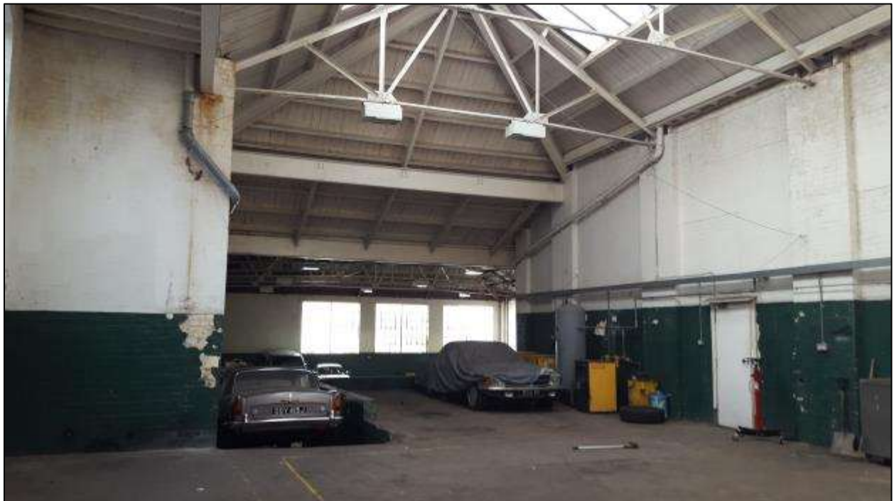
Figure 10: Inside the eastern workshop.
