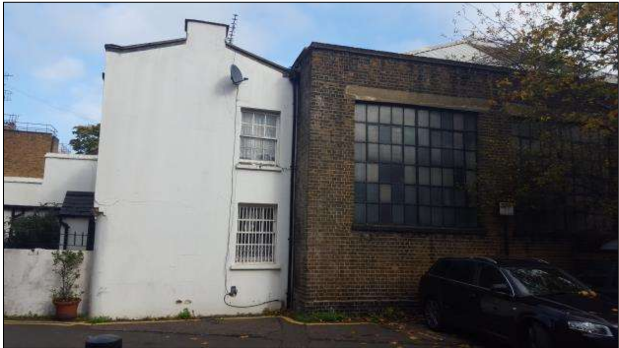
Figure 3: The southern elevation of B1.
