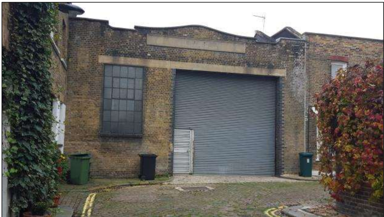
Figure 6: The eastern elevation of B1.
