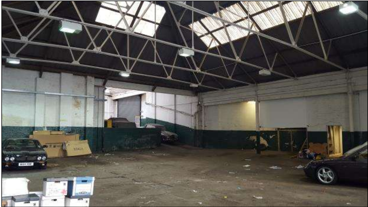
Figure 9: Inside the eastern workshop.
