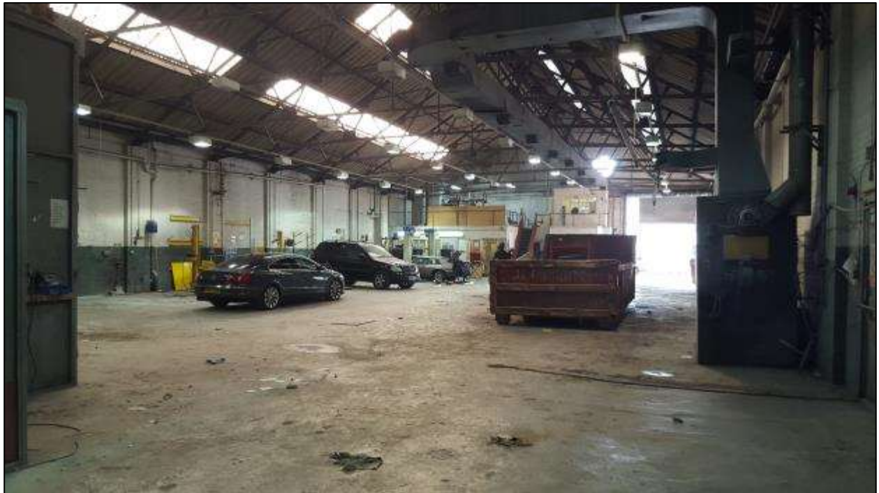
Figure 8: interior of the western workshop of B1, looking south.
