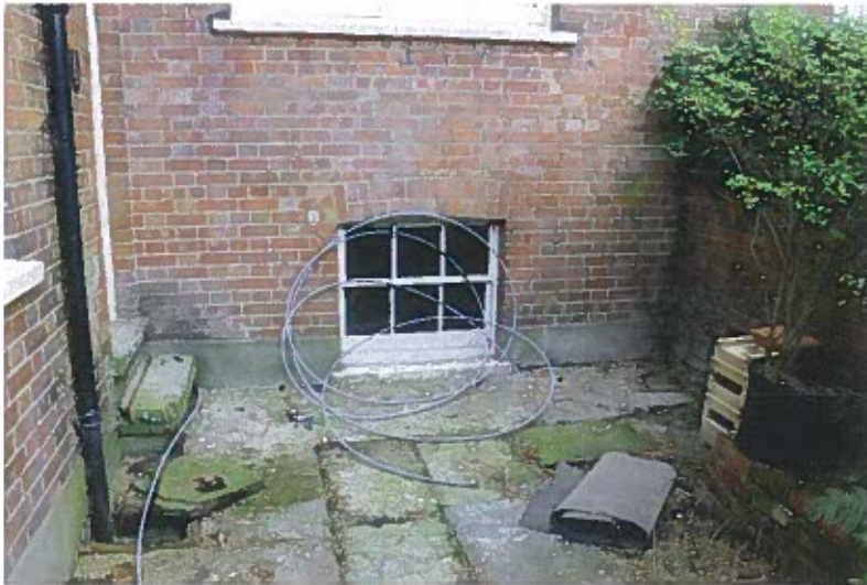
Existing basement window to be replaced
