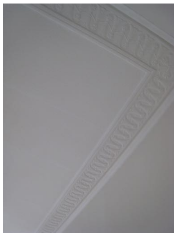
front bedroom - restored cornice
