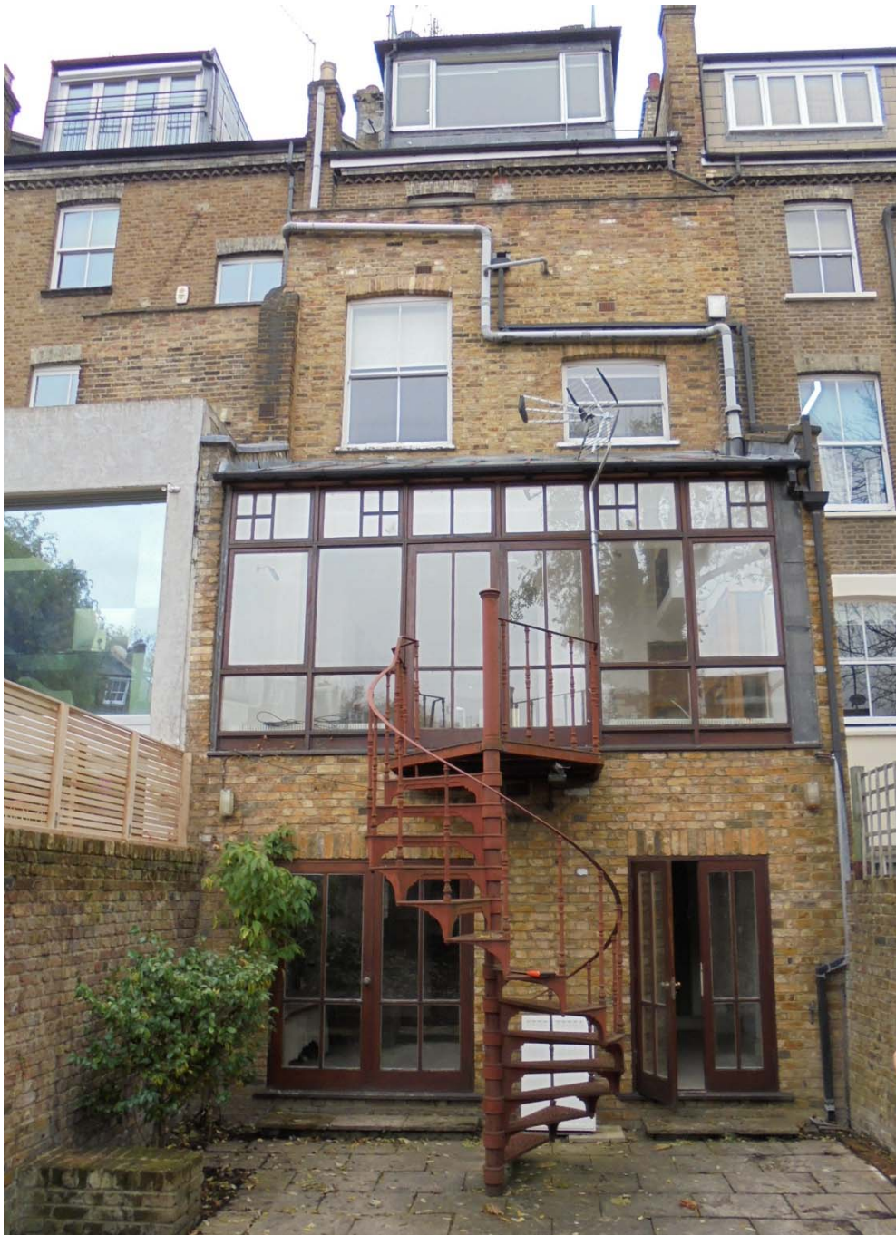
Existing photograph of the rear of the property
