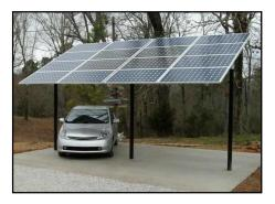
10m<sup>2</sup> for polycrystalline panels will generate 1kWp(kWp-energy generated at full sunlight) of electricity.
