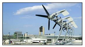
10 kW. For isolated grid applications, the turbines are typically larger, ranging from about 10 to 200 kW. Wind turbines are mounted on a tower to harness the most energy. At 30 meters or more aboveground, they can capture the faster and less turbulent wind in an urban environment. Turbines harness the wind's energy with their propeller-like blades. In most of the cases, two or three blades are mounted on a shaft to form a rotor.
