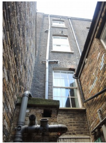
12 Argyle Square rear elevation
