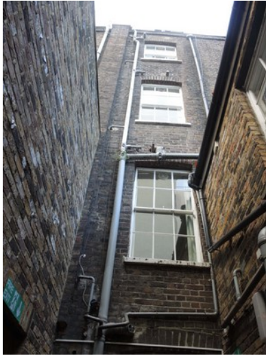
11 Argyle Square rear elevation
