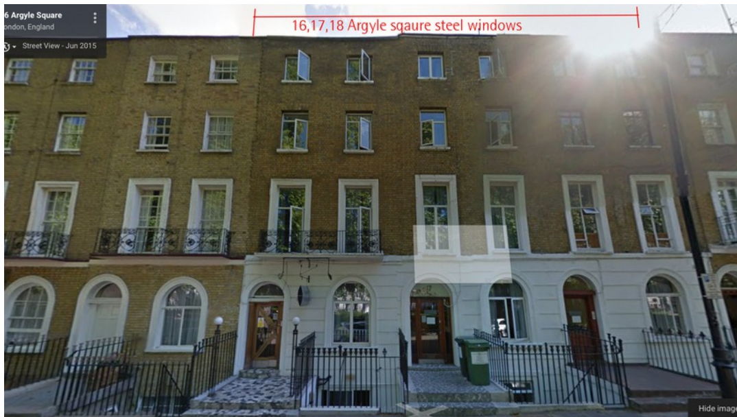
16,17,18 Argyle square with steel windows
