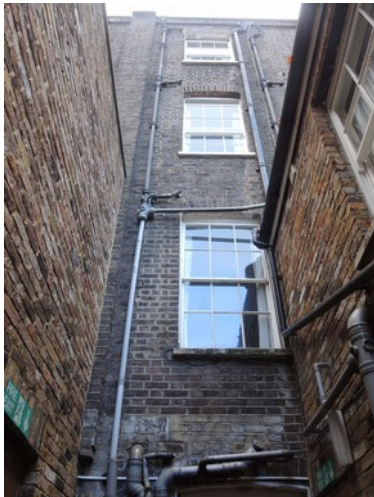
13 Argyle Square rear elevation
