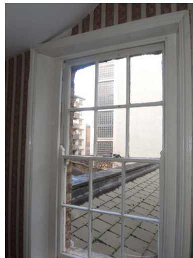
15 Argyle Square rear window internal view at Stairwell
