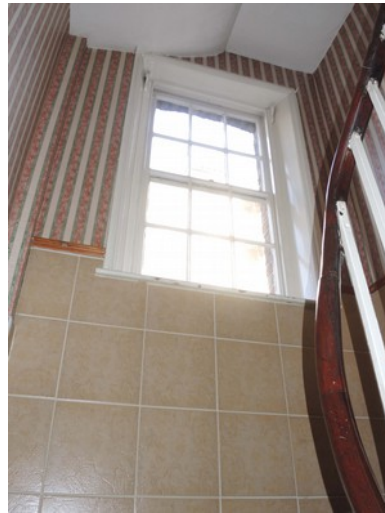
13 Argyle Square rear window internal view at Stairwell
