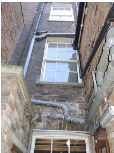
15 Argyle Square rear elevation
