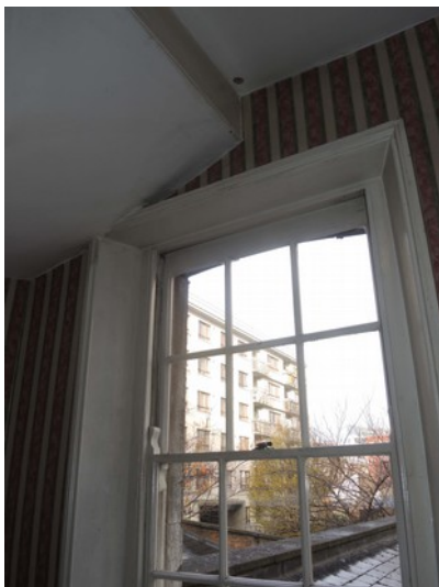
14 Argyle Square rear window internal view at Stairwell
