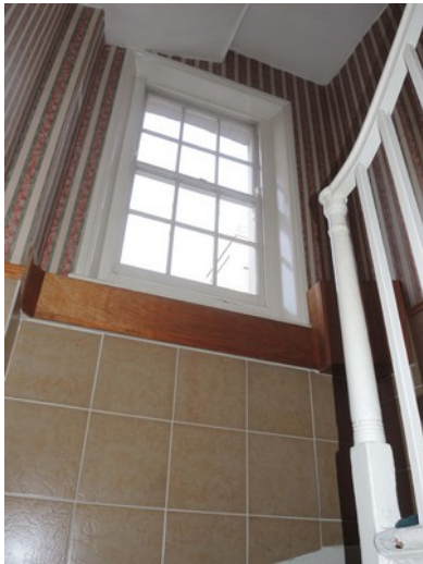
12 Argyle Square rear window internal view at Stairwell
