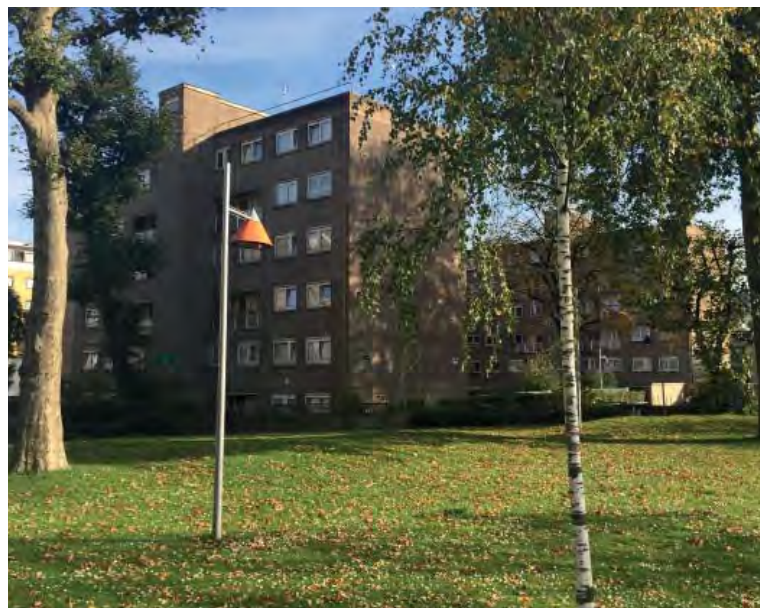
Fig 6: Mid rise residential blocks adjacent to the site
