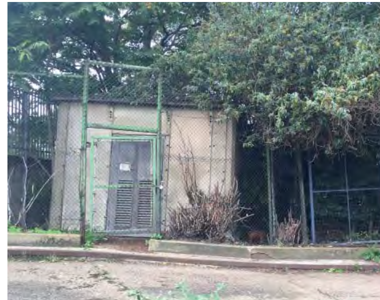
Fig 11: Street view of Substation building.
