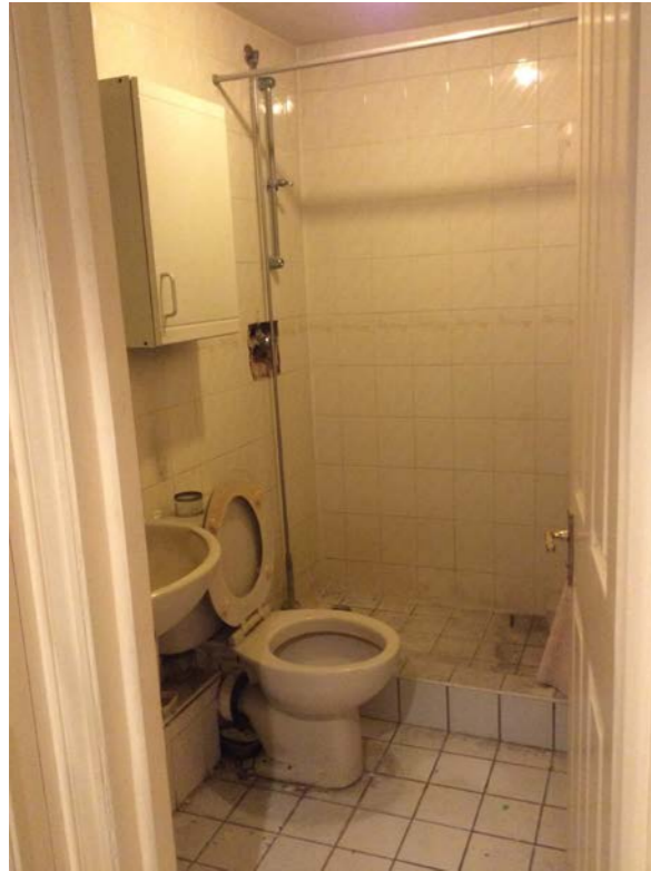
Fig 1: Existing en-suite shower room
