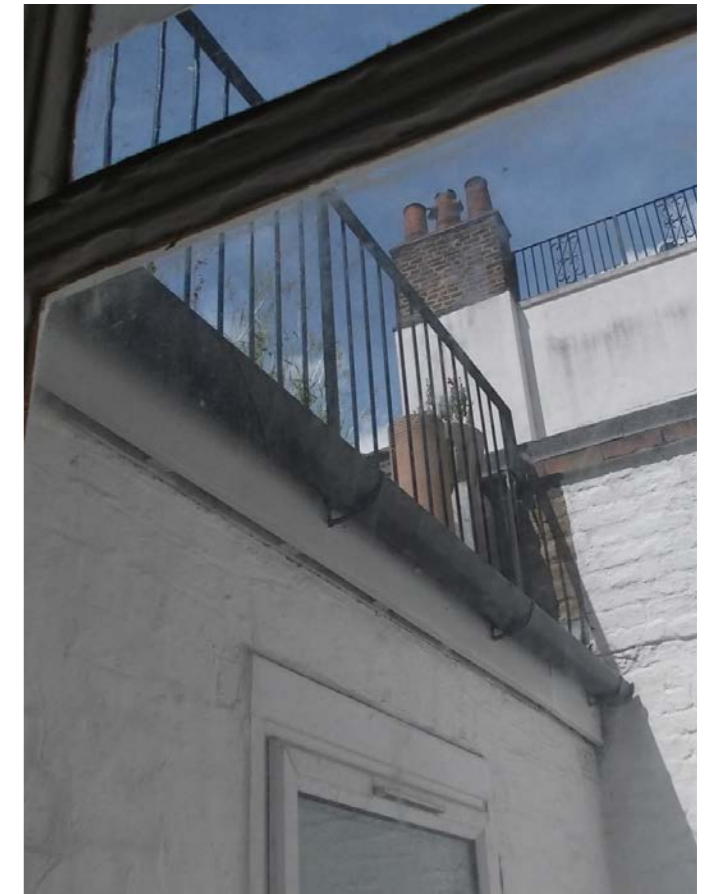
Fig 4. Gutter to 1st floor rear terrace
