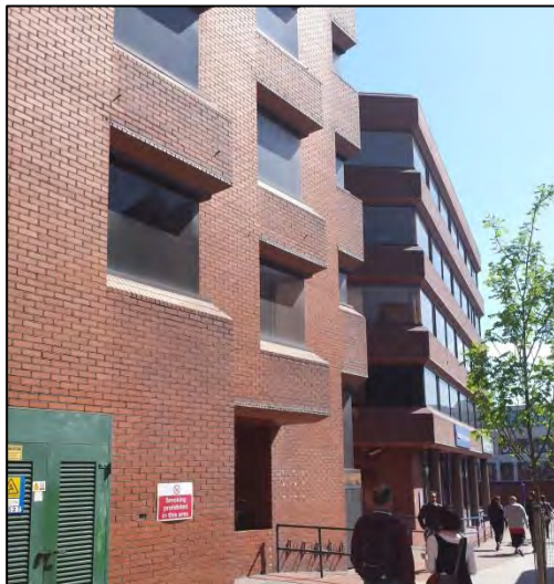
Figure 3: 'Northern' Council Offices of the site. Viewing ~ SE
