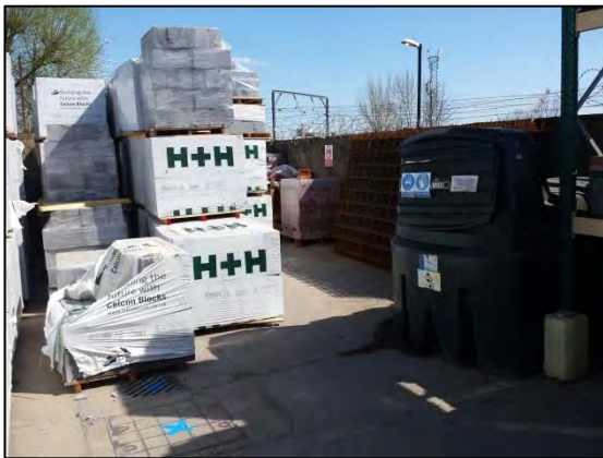
Figure 40: 2500L Diesel storage tank in south eastern corner of the site, visible staining at base. Viewing ~SE
