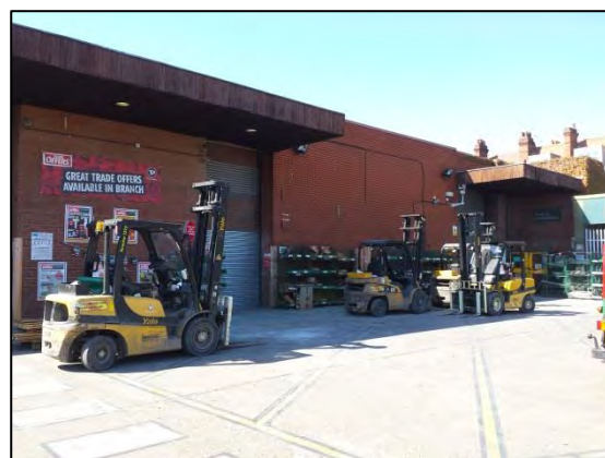
Figure 47: Forklift storage/parking area adjacent to main building. Viewing ~ NW
