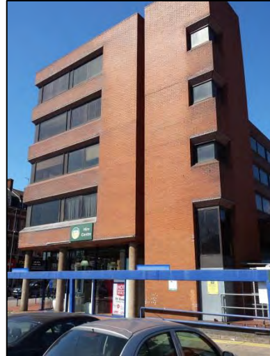
Figure 2: Ground floor Wickes and above office space. Viewing ~ NW
