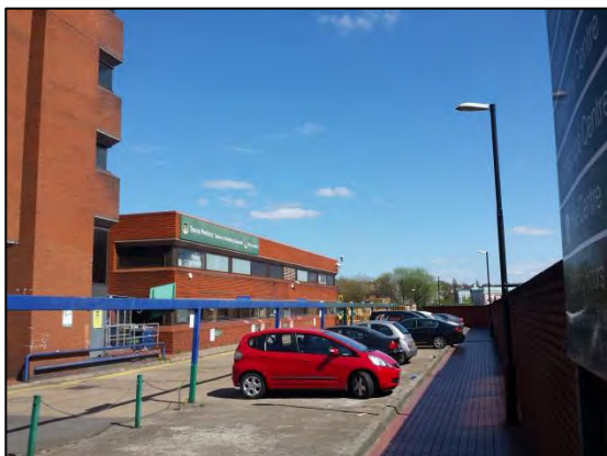
Figure 7: Car Park area and public footpath adjacent to southern boundary. Viewing ~ NE
