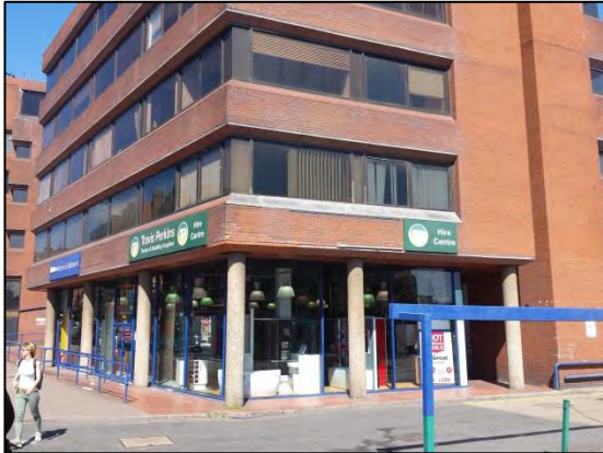
Figure 1: Ground floor Wickes showroom with offices above. Viewing ~ NE
