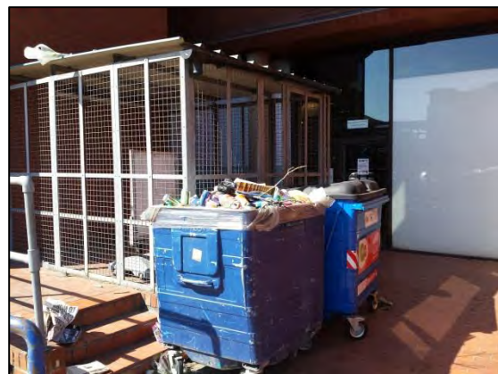
Figure 6: Metal storage cage and waste bin storage area
