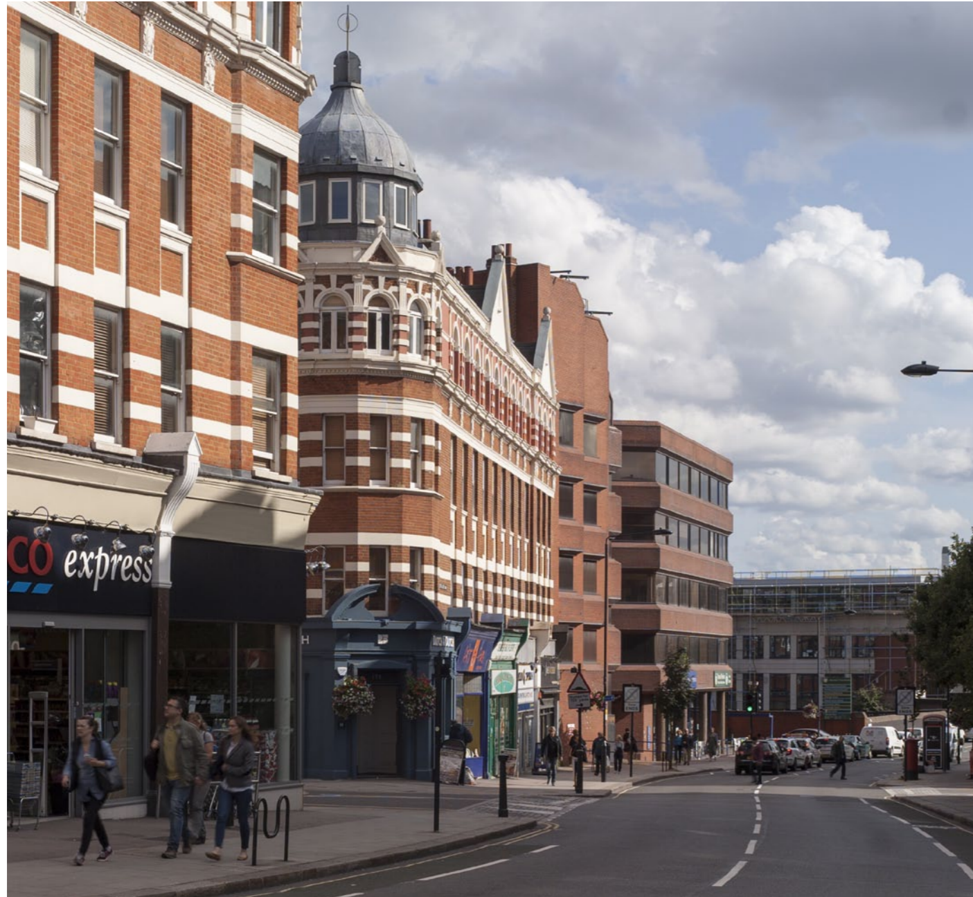
View looking south along West End Lane - As Existing
