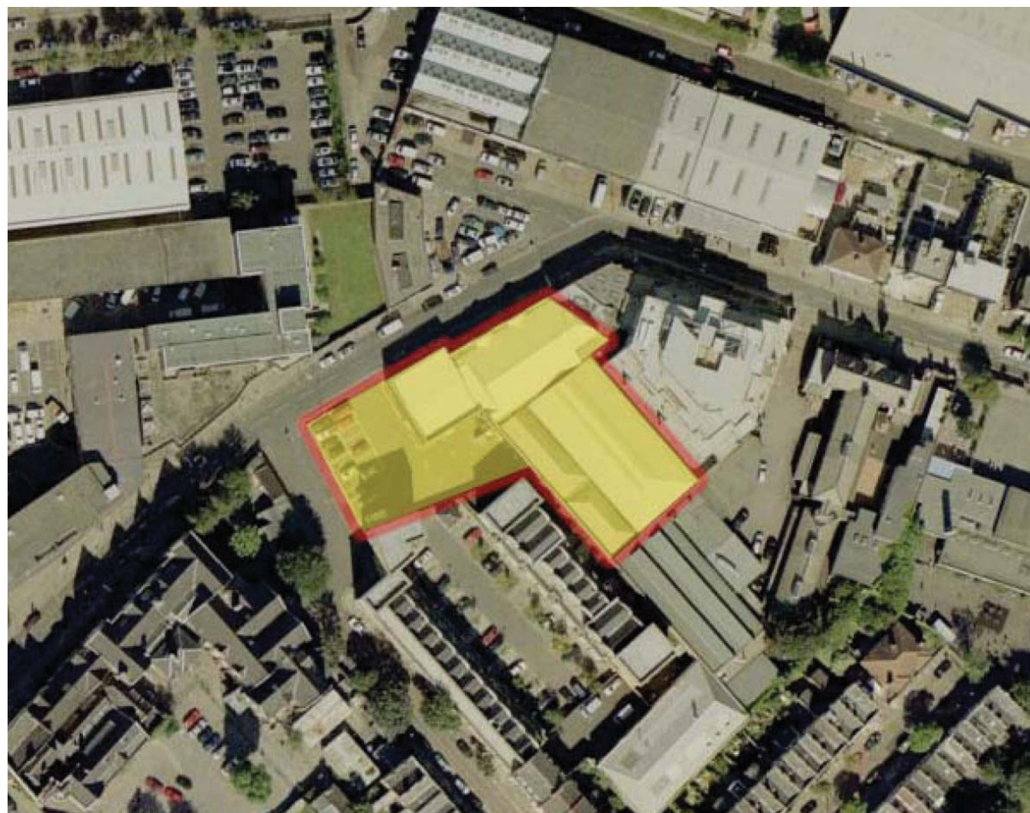
Aerial Photograph Showing Site Location
