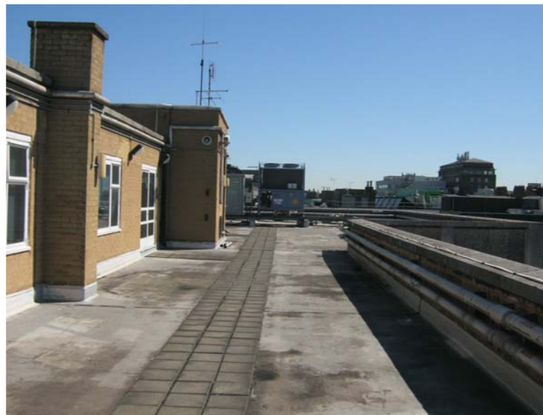
View of Existing Roof
