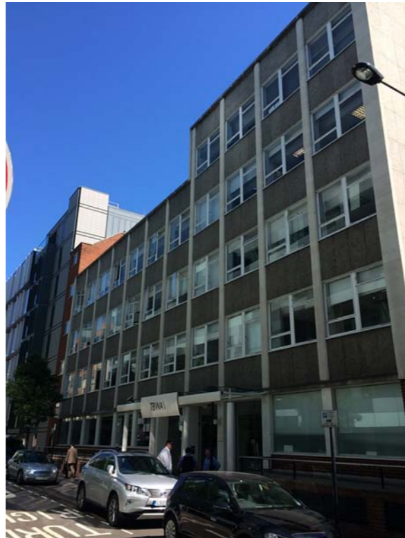
North approach on Whitfield Street
