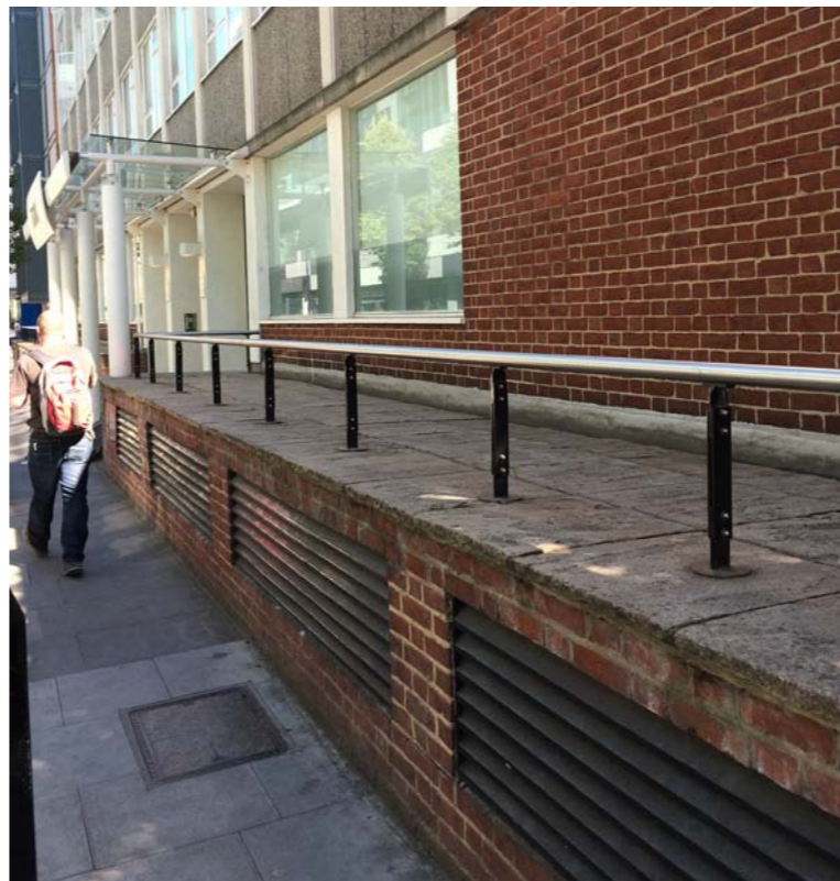
Existing brick plinth & entrance
