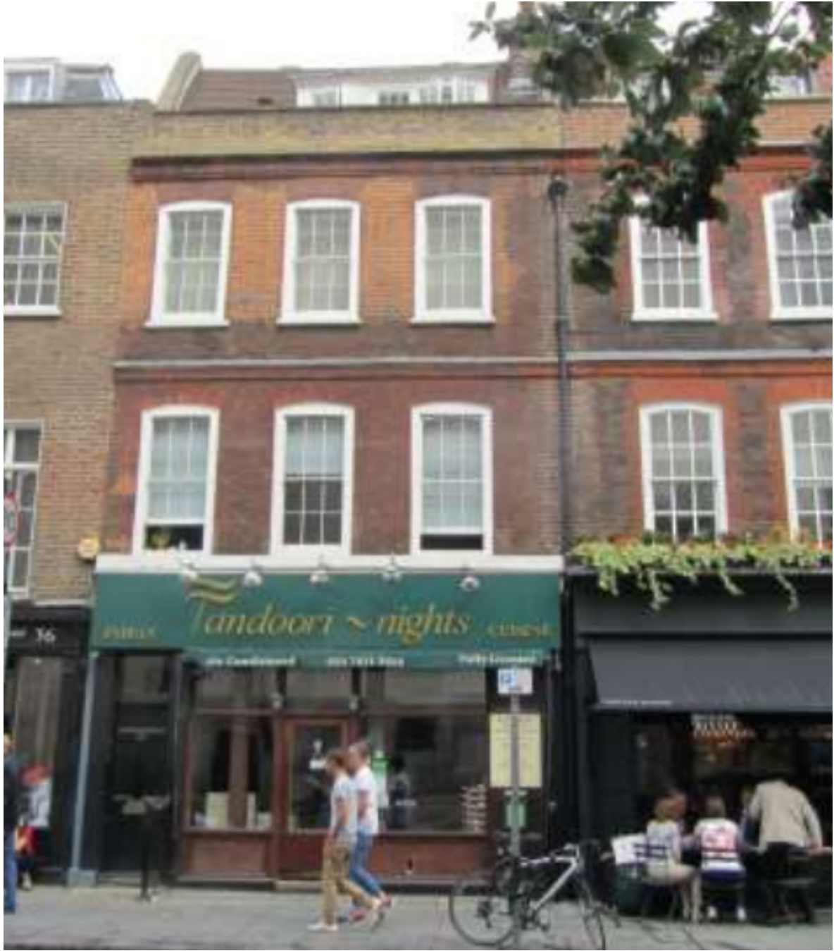
Photo 5: Front elevation of host building
