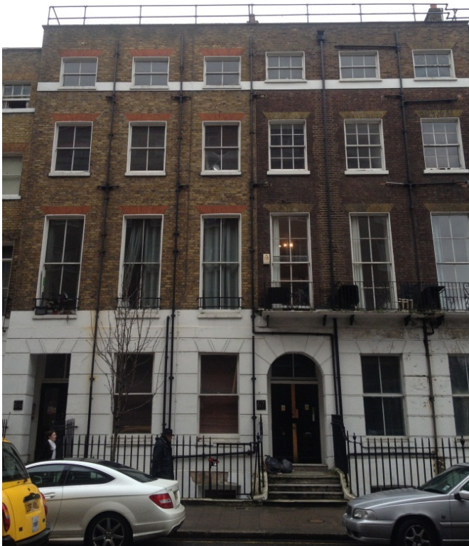
Figure 1: No. 66 Guilford Street, main elevation.
