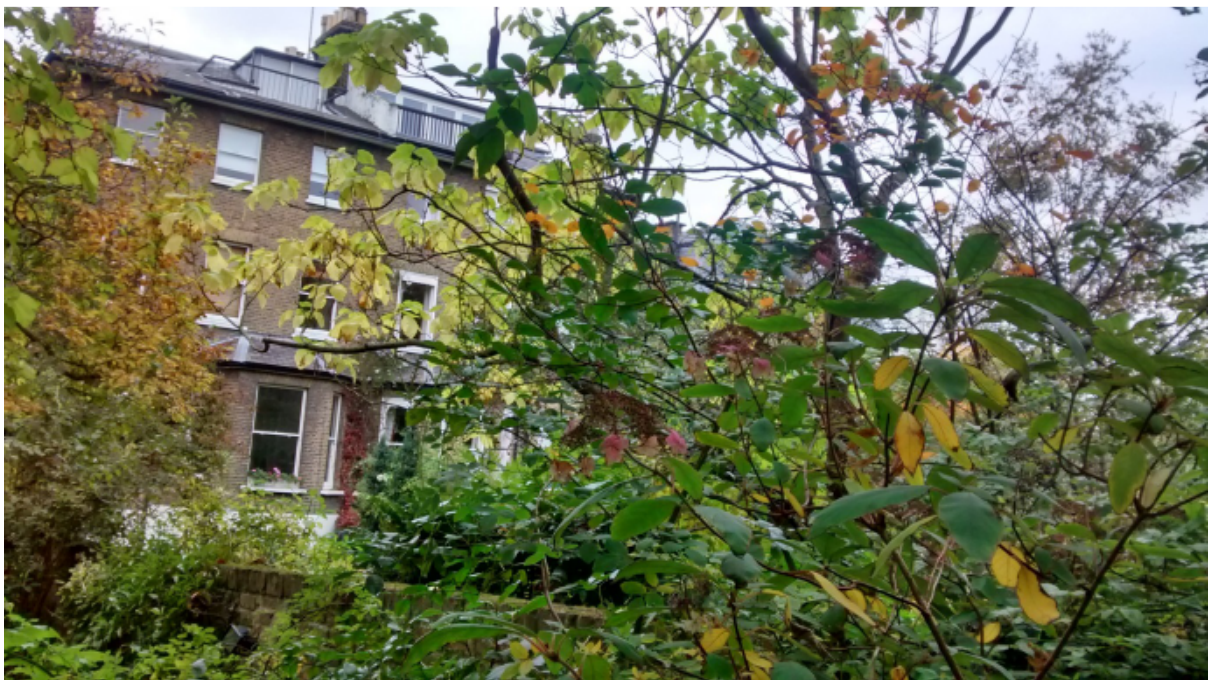
4. Looking east towards no. 11 Elsworthy Road
