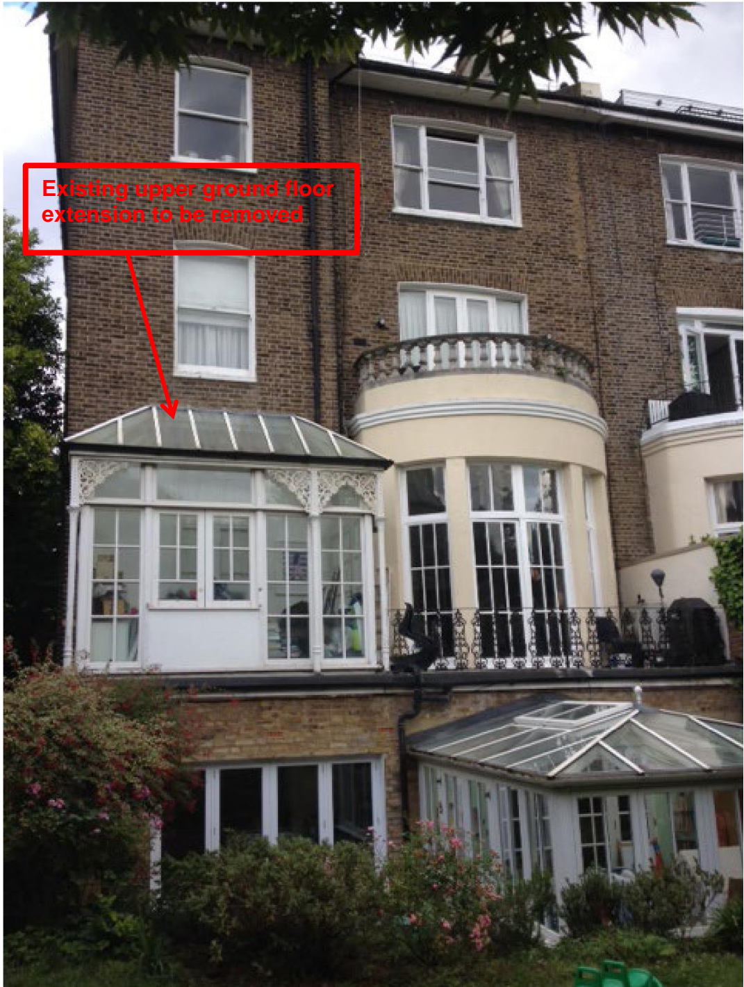
Photo 1- Existing rear elevation
