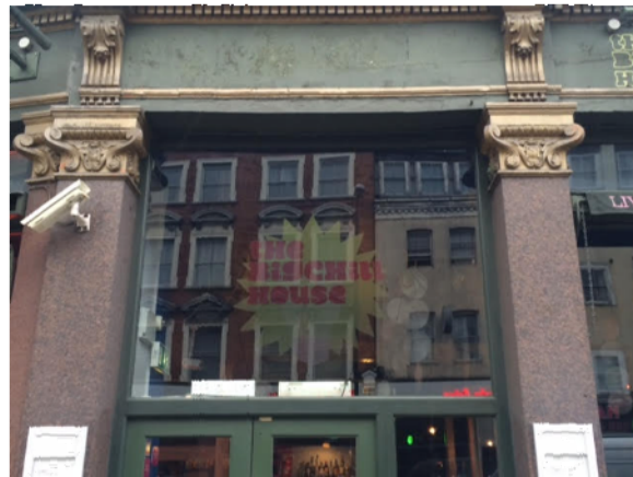
EXISTING VINYL SIGNAGE BEHIND GLASS PANEL
