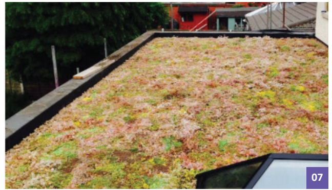
07 Example of a variegated sedum roof
