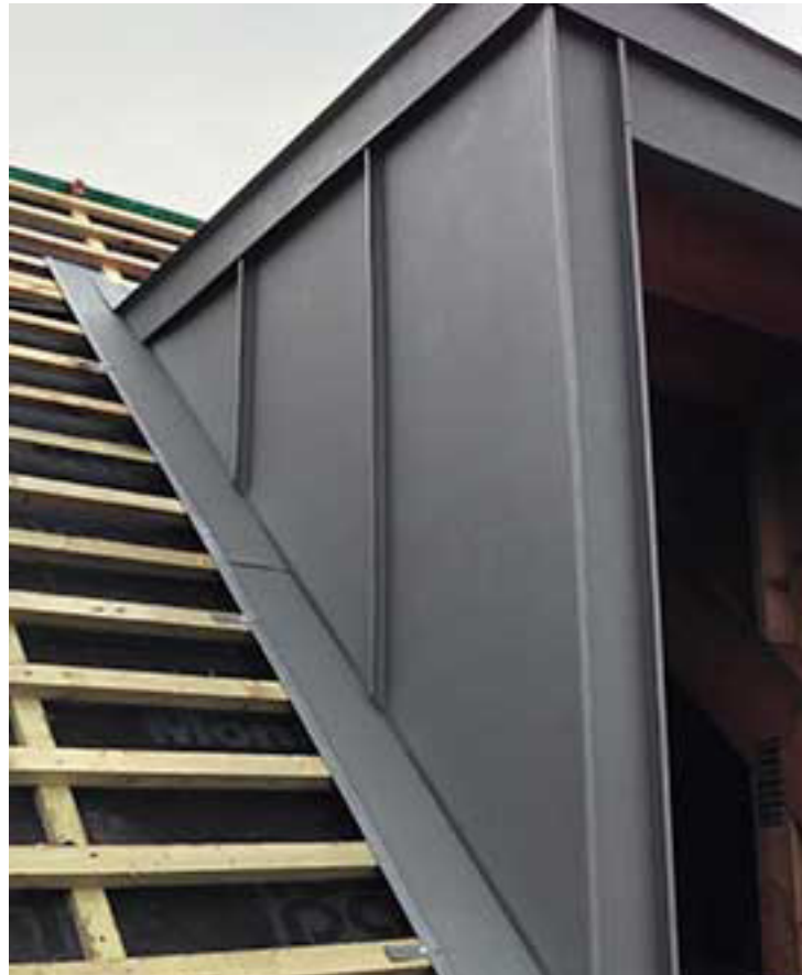
Natural Zinc cladding for Roof Extension
