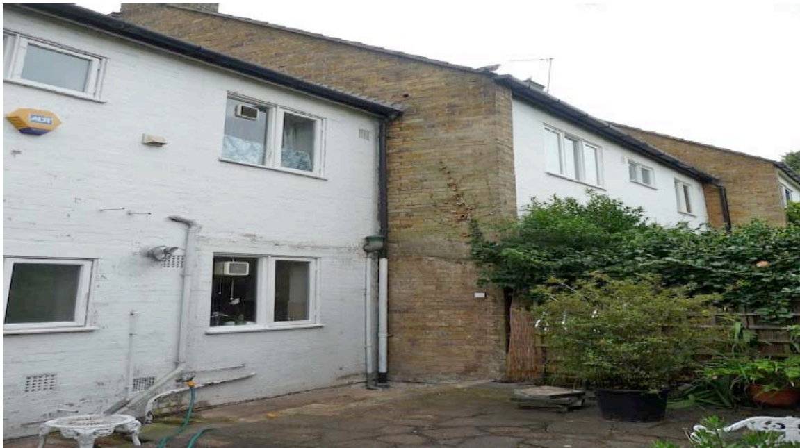
Rear View of 35 Rudall Crescent
