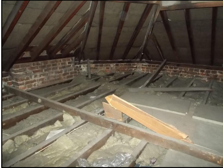
Fig. 10: Existing View – Roof void
