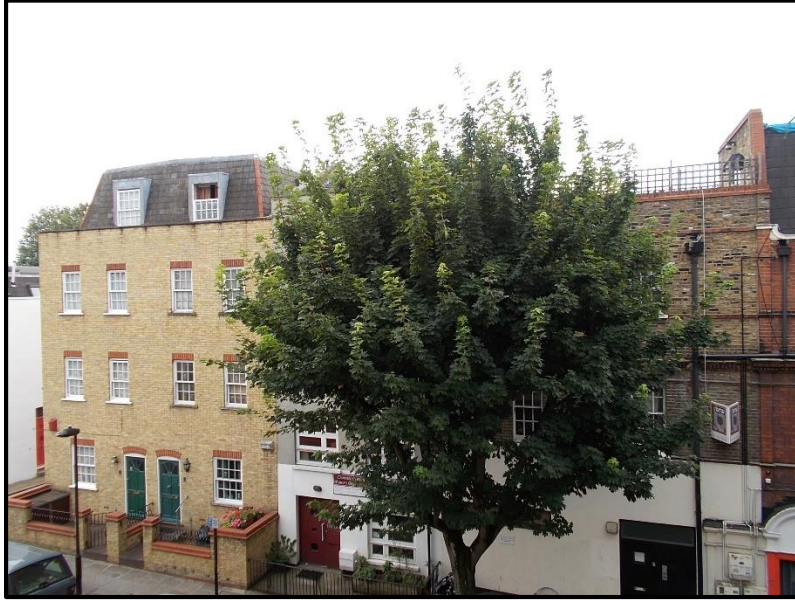
Fig. 12: Neighbouring residential building along Falkland Road supporting a Mansard style roof as existing
