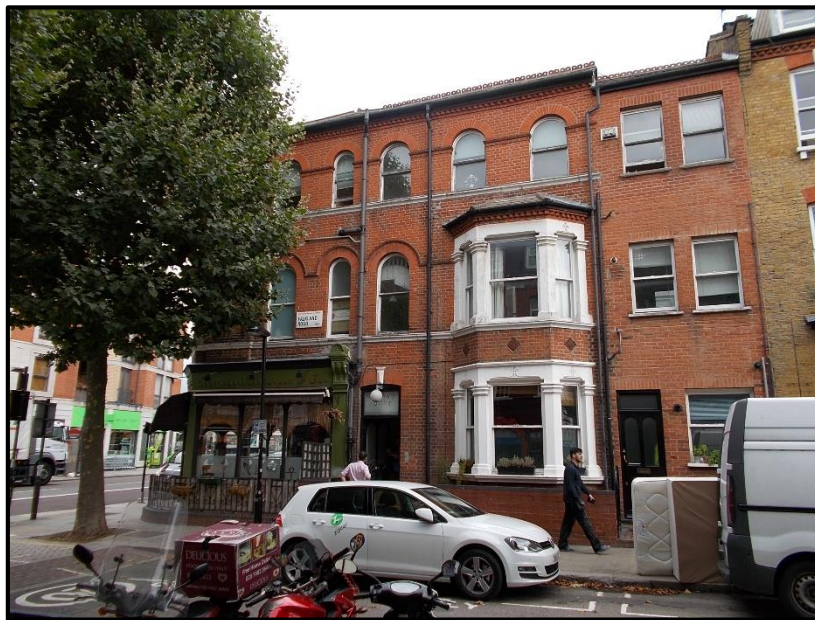
Fig. 7: Existing View - The application building from Falkland Road
