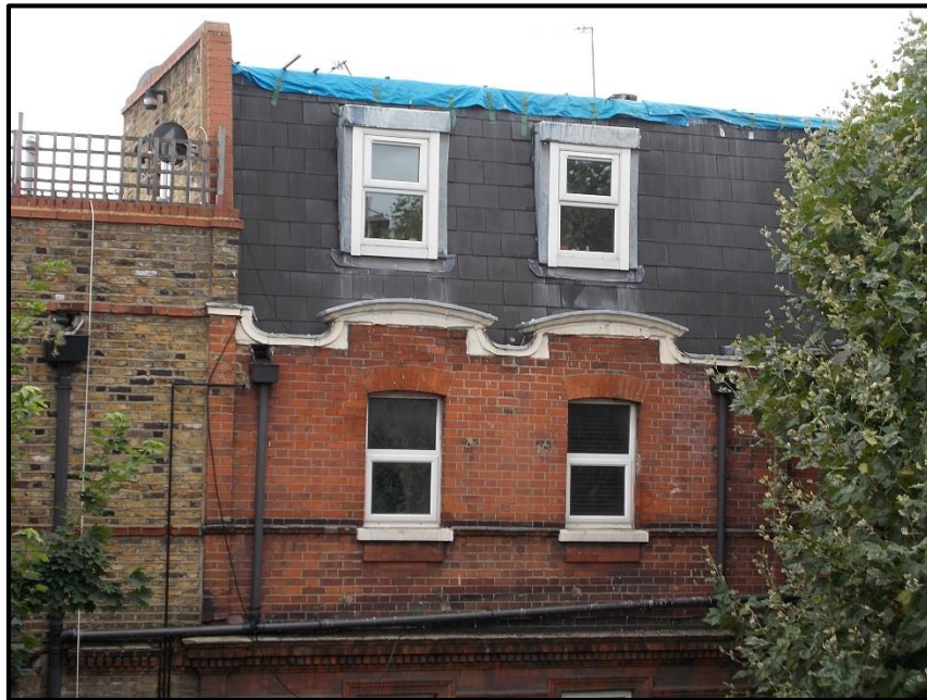
Fig. 13: Neighbouring residential building along Falkland Road supporting a Mansard style roof as existing
