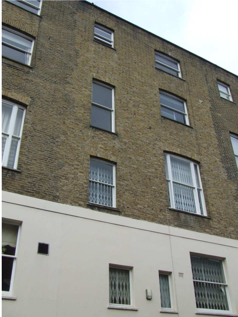
Existing rear elevation of number 33, showing the existing single glazed units
