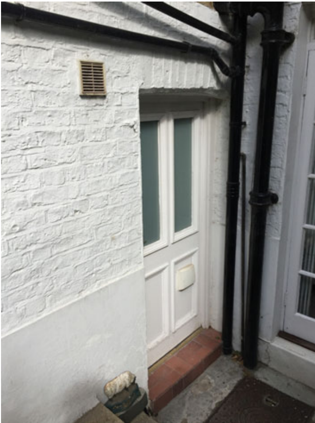
Door in closet wing
