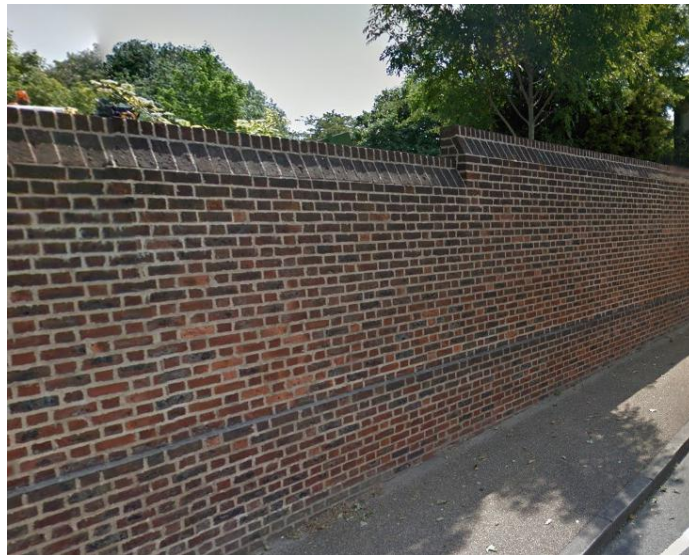
Photograph 9: Existing Listed boundary wall to site
