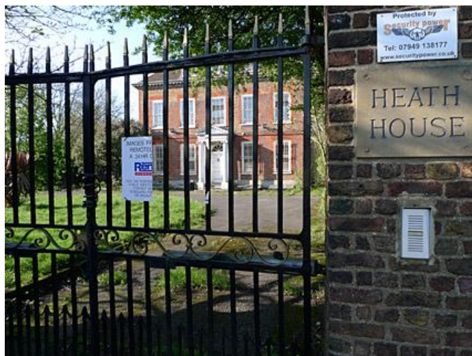
Photograph 10: Existing Wrought Iron gates to Heath House
