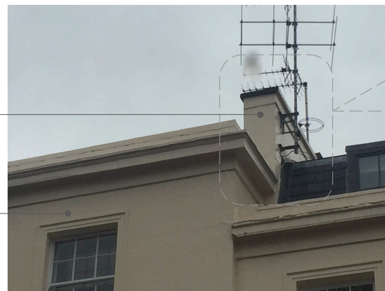
Image of existing chimney breast along party wall
