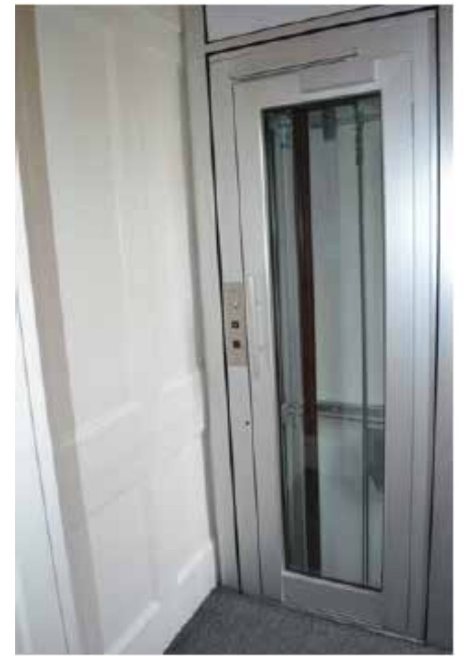
Fig.16 - Lift insertion
