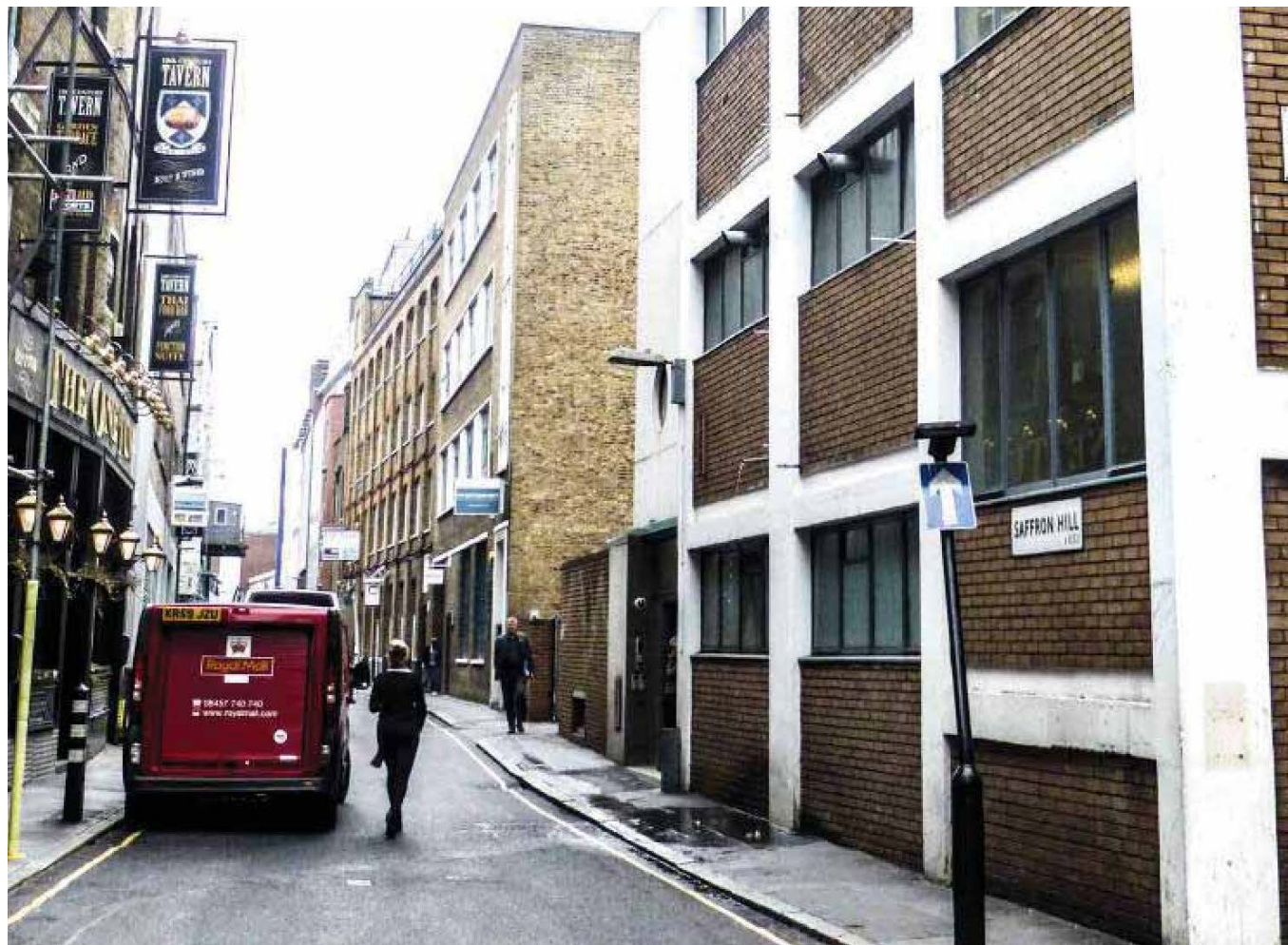
Left: View down Saffron Hill from Greville Street. 29-35 Farringdon Road is to the right of the picture with the application site behind it.
