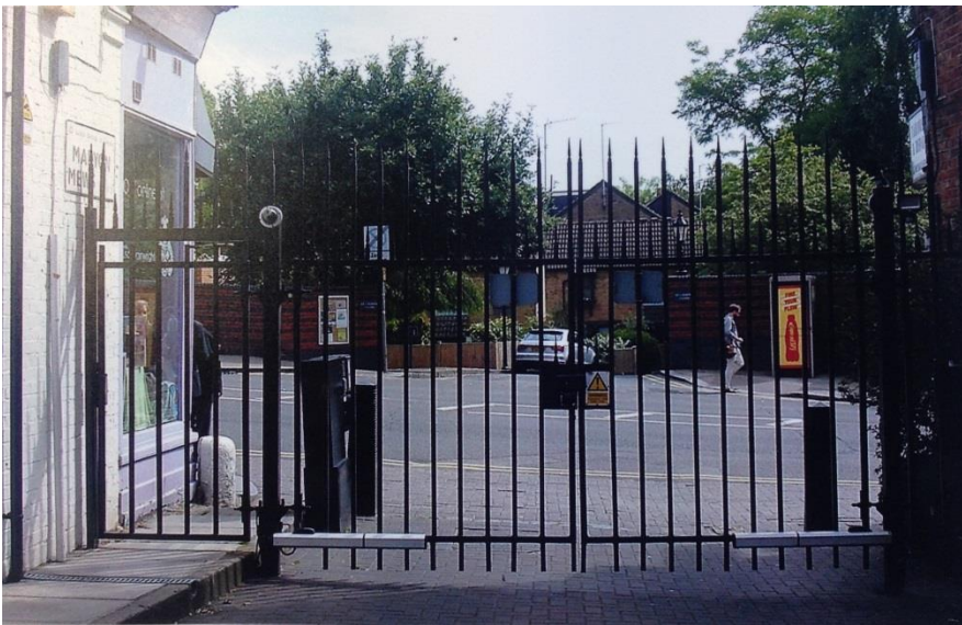
Figure 1: North Entrance to Maryon Mews looking from the Mews onto South End road
