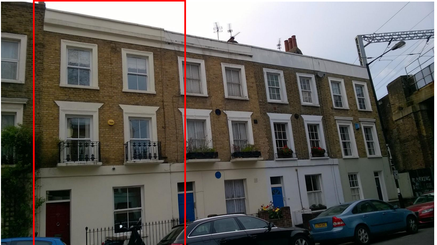
Figure 7 – (Right- looking towards Railway Bridge) Site front elevation
