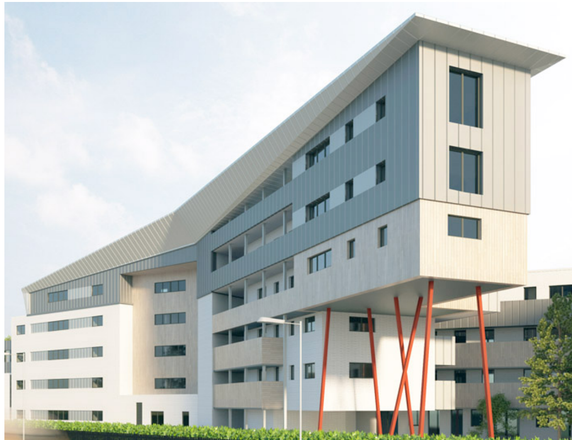
VIEW FROM THE WEST END OF WEST HAMPSTEAD STATION
