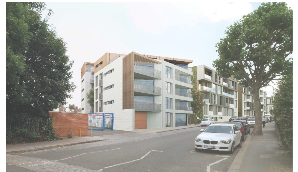
159-161 IVERSON ROAD (CURRENTLY UNDER CONSTRUCTION) INFRONT OF APPLICATION SITE
