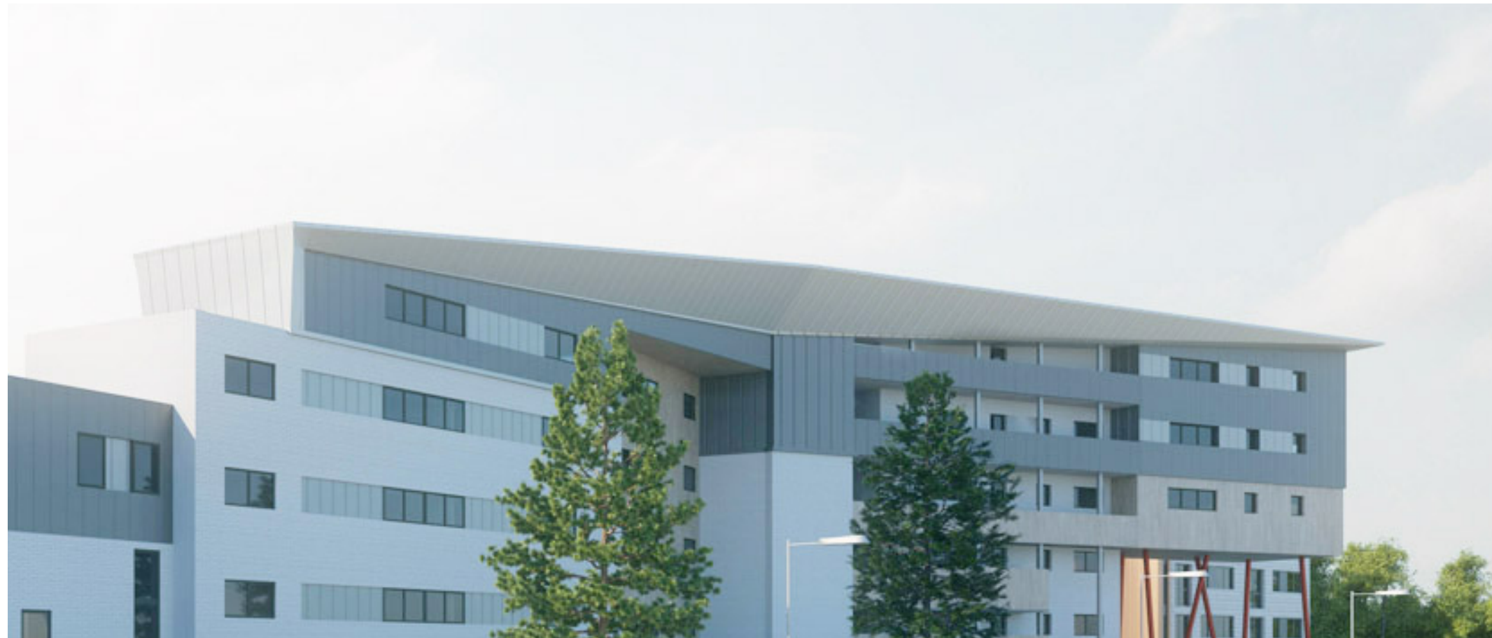
VIEW FROM THE EAST END OF WEST HAMPSTEAD STATION
