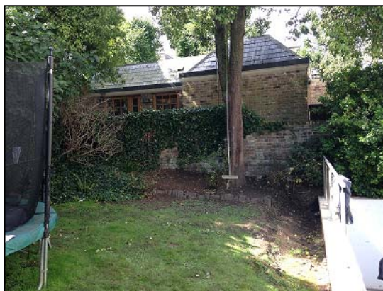
View of the area behind the top retaining wall.
