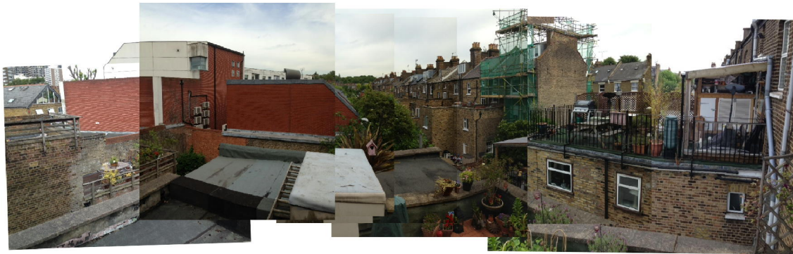
PHOTOGRAPH 3 - Composite panorama photograph showing the blank flank walls of the commercial buildings in Heatgate Place immediately to the rear of 8 Mansfield Road and the neighbouring rear roof terraces at 4 and 10 Mansfield Road.
