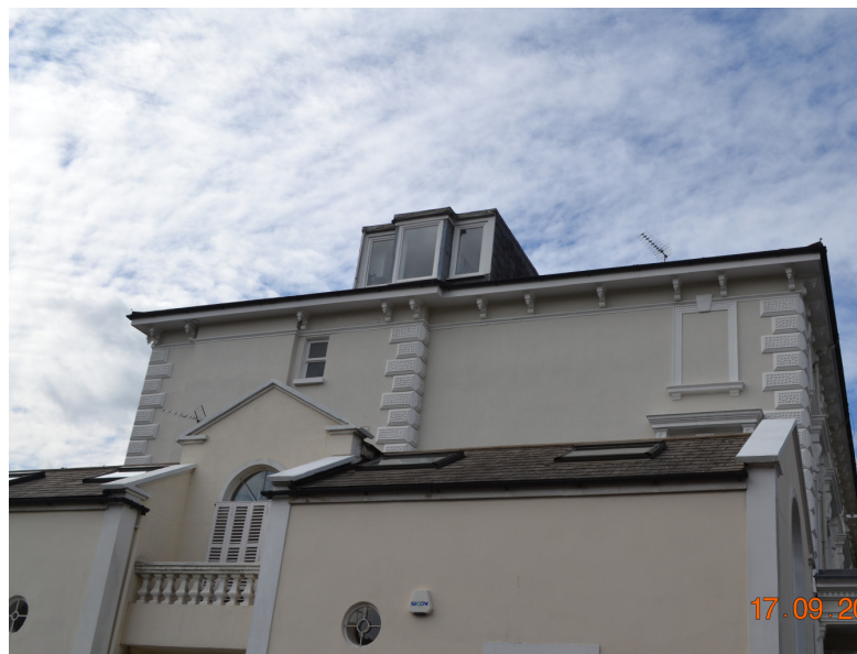
External side elevation of existing third bedroom door.
