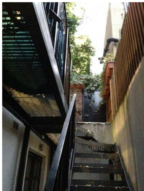
Photo 3 Flat 2 no. 17 Existing terrace and stair
