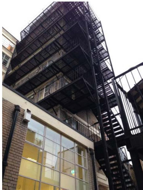
Photo 1 neighbouring property west of the light well/alleyway
