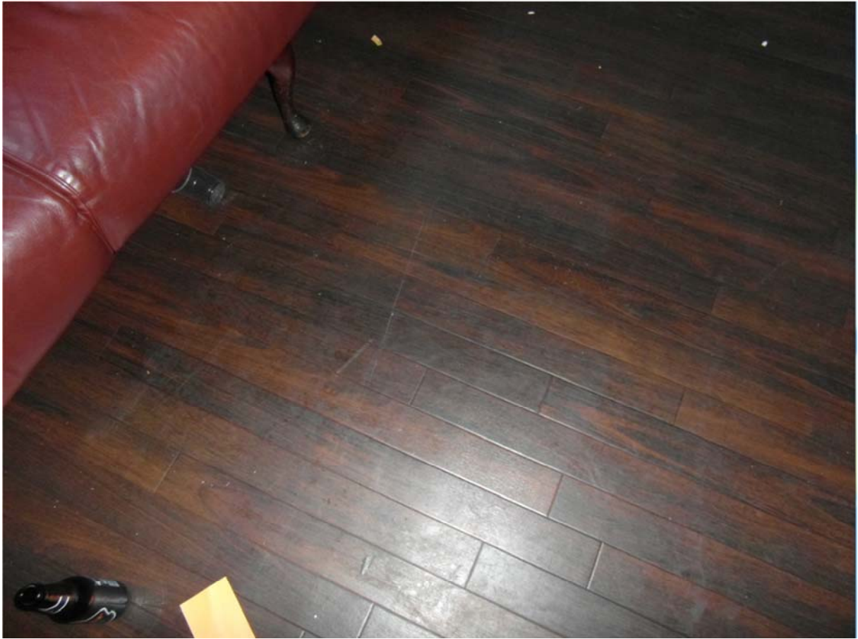
First Floor Non-Original Flooring
