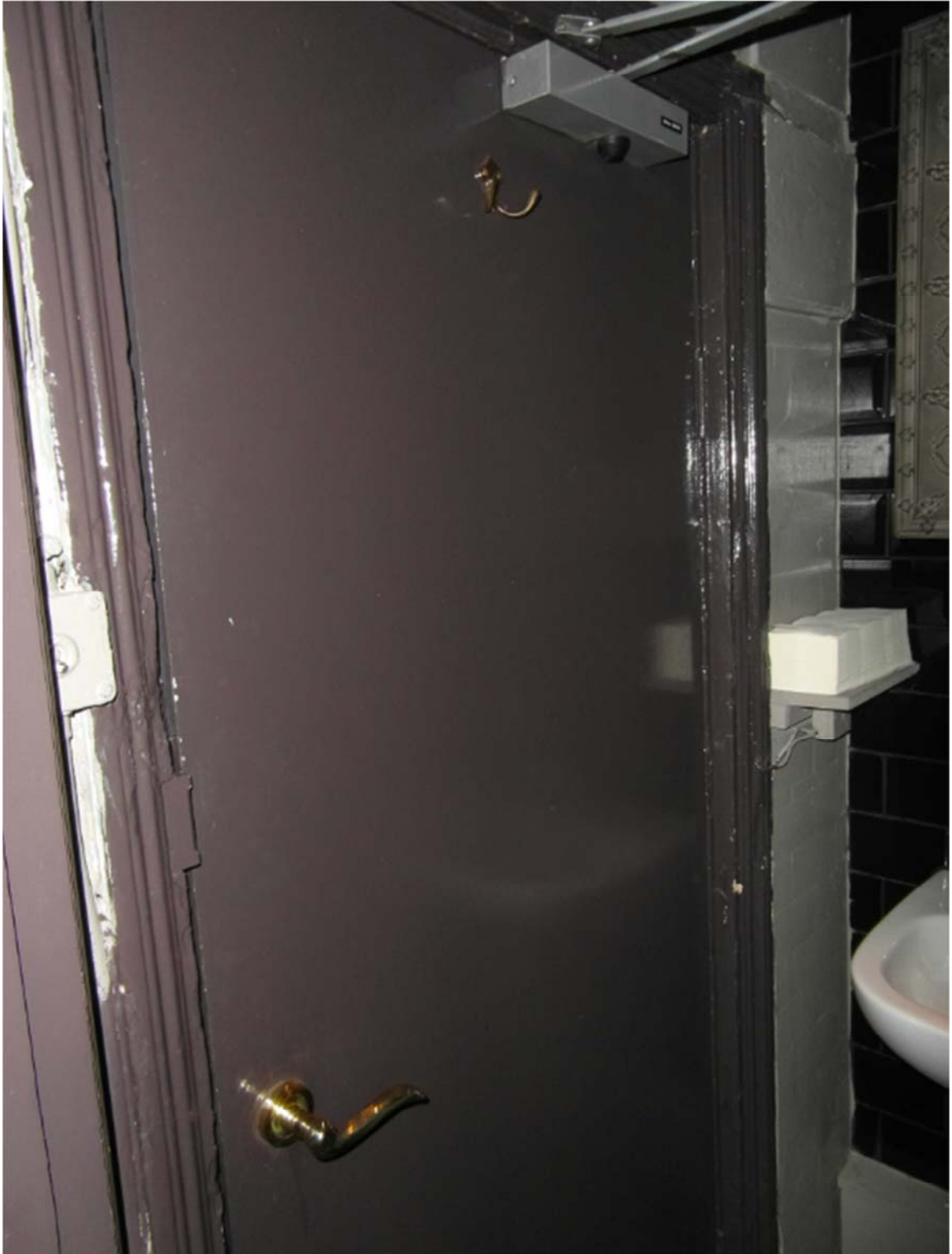
Third Floor Bathroom Door 1
