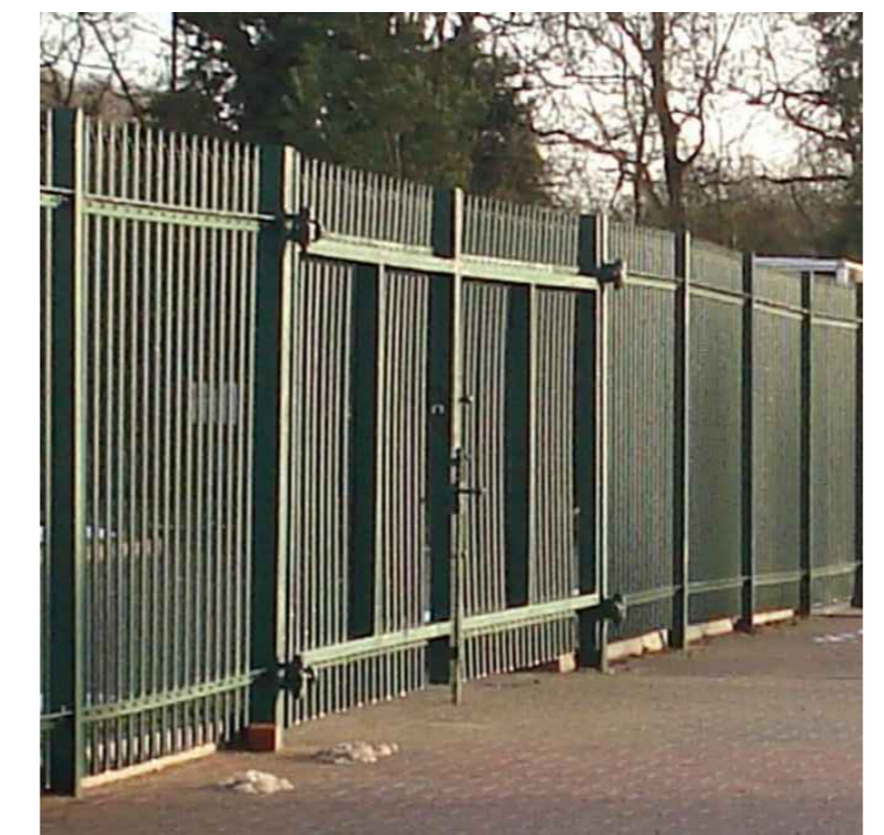
2. Proposed 1m width x 2.4m high Barkers ProtectorGate single leaf pedestrian gate. Type and finish to match existing as shown in image 1.
