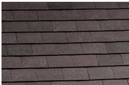
Clay tiles roofing material- matching as existing
