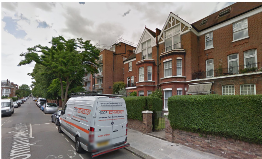
Front elevation of 72 Compayne Gardens and rest of the terrace
