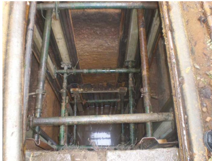
Figure 3 Propping
