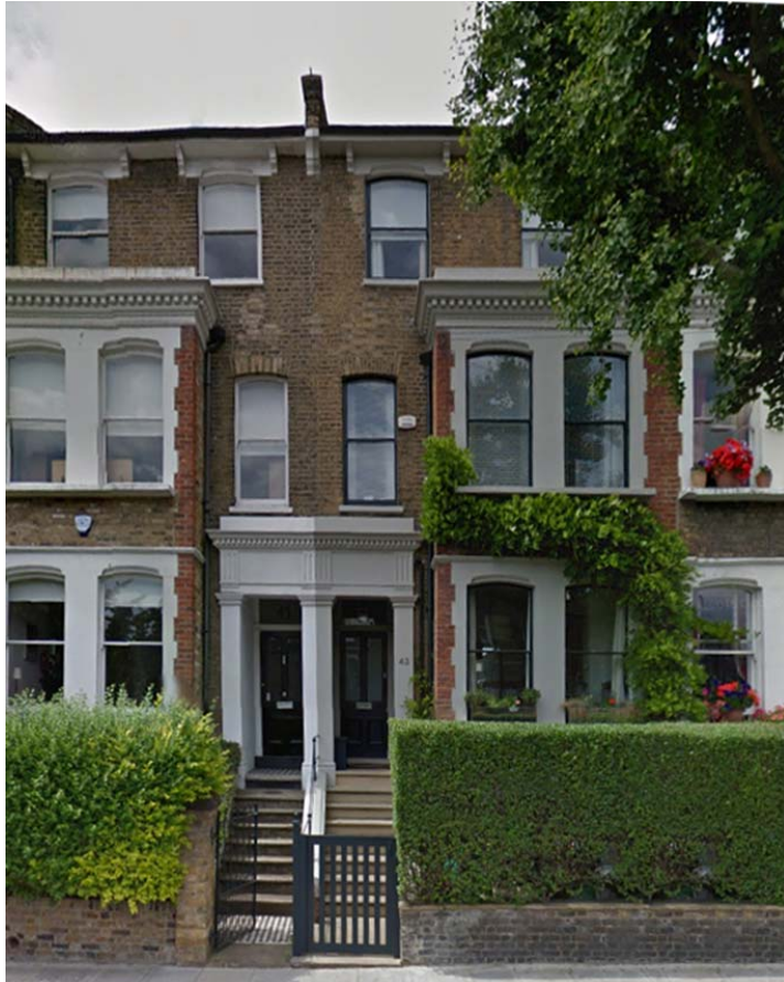
the front of the property
