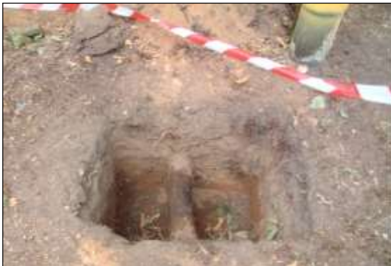
Photo 38: Where piles are proposed close to trunks, it is essential to excavate 50–75cm deep to see if there are any significant roots in the way, with provision to move the pile location if roots are found (note the pile was finally installed to avoid this root).
