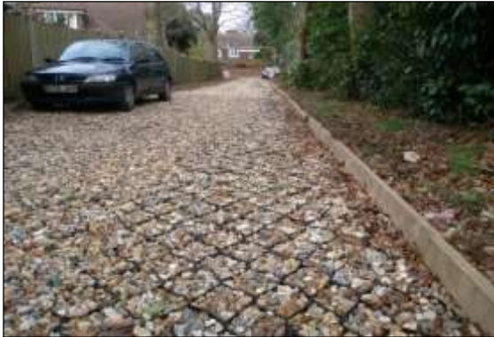
Photo 28: Wooden board pinned in place or held in position with backfilled topsoil can provide more informal and rustic surface edging.
