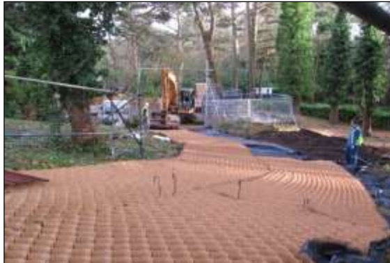
Photo 24: The three-dimensional cells are opened up, spread across the area to be surfaced and pinned in place ready for the stone filling.
