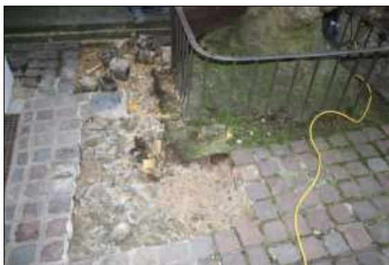
Photo 21: Careful lifting of cemented-in sets round this tree allowed them to be re-laid on a permeable sand base, improving the water input into the soil around the trunk.
