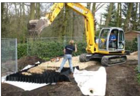
Photo 11: Cellular products are a very effective means of providing ground protection where heavy vehicle use is expected. Here, it is being used to temporarily widen an existing road, to be removed once the construction is finished.
