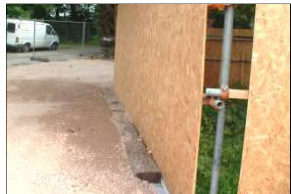
Photo 27: Although this is only a temporary surface, railway sleepers pinned into the ground can be used to retain the edges of new surfacing.
