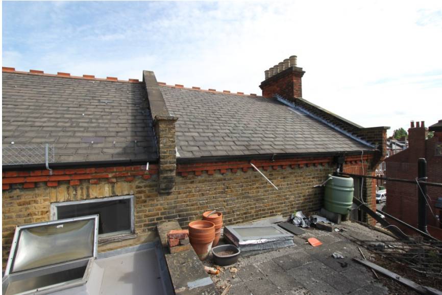
9. Rear view of 86 (LHS) and 88 (RHS)
