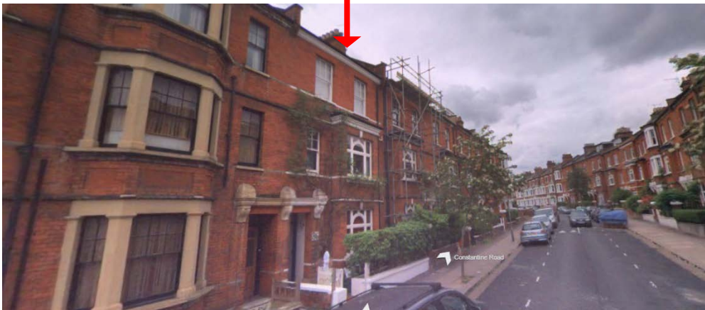
4. View of 86 Constantine Road looking south
