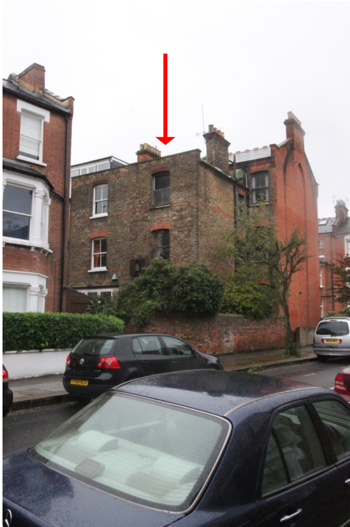
6. Rear view of No. 84, 86 and 88 from Mackeson Road demonstrating how the proposed dormer and terrace would be largely concealed from view (No.84 dormer is only partly visible)
