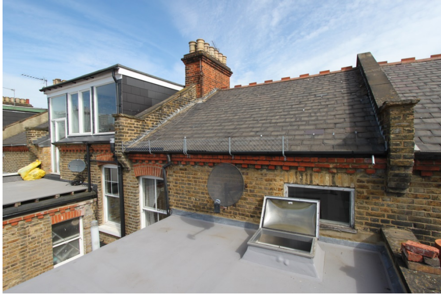
8. Rear view of 84 (LHS) and 86 (RHS)
