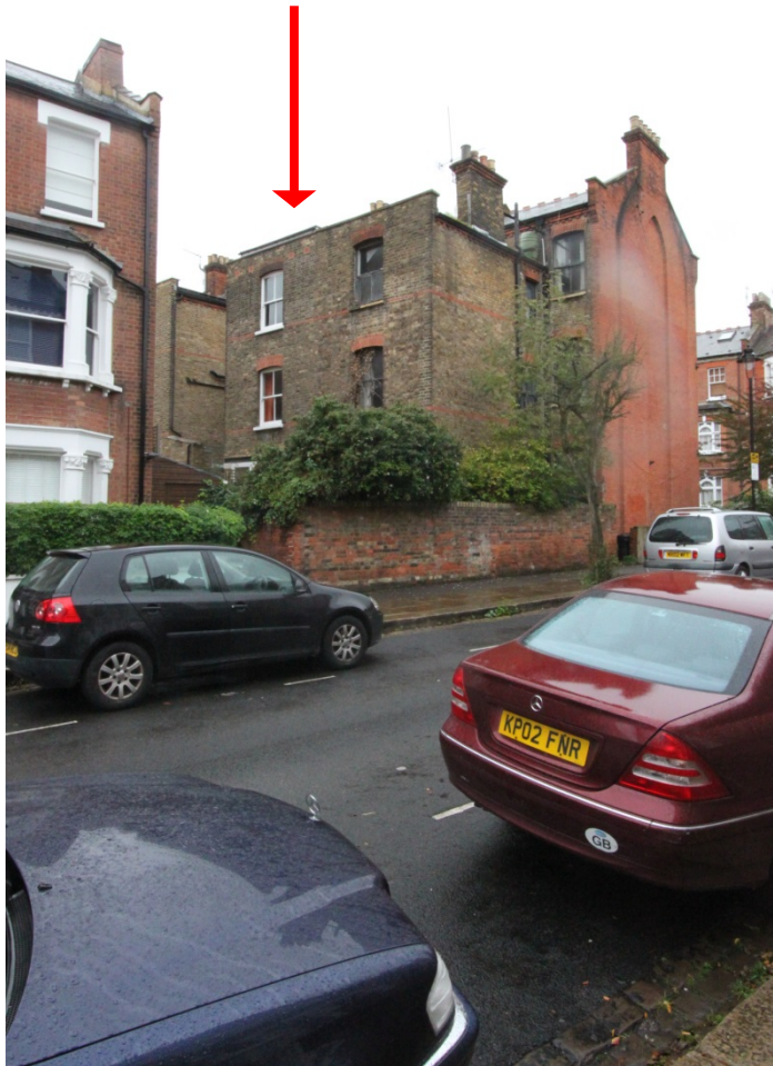
5. Rear view of No. 84, 86 and 88 from Mackeson Road demonstrating how the proposed dormer and terrace would be largely concealed from view (No.86 below arrow)
