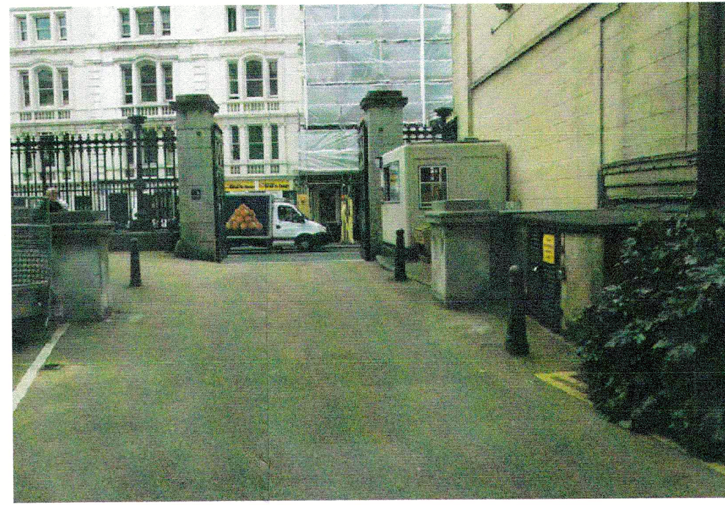
EXISTING GATE (VIEW FROM INSIDE PERIMETER)
