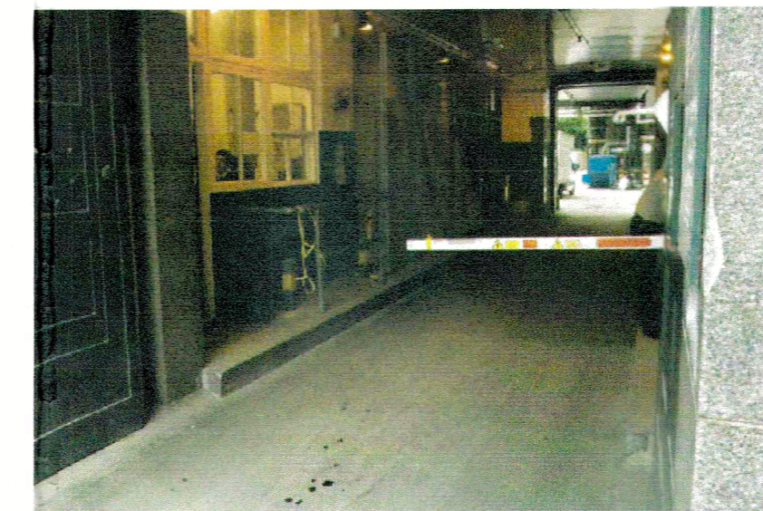
EXISTING NORTH EAST GATE (VIEW FROM OUTSIDE PERIMETER)
