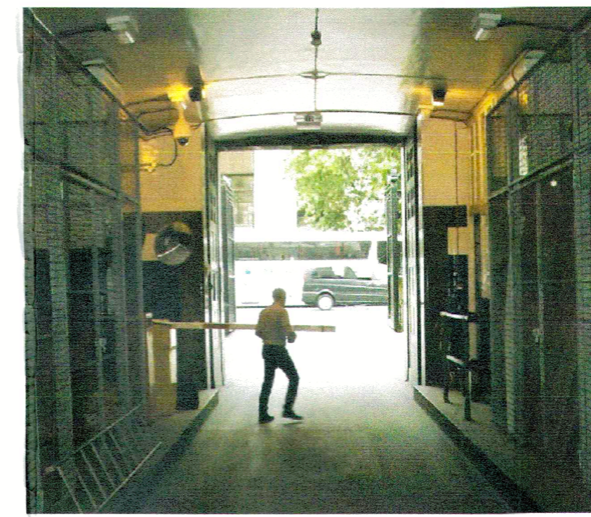
EXISTING NORTH EAST GATE (VIEW FROM INSIDE PERIMETER)
