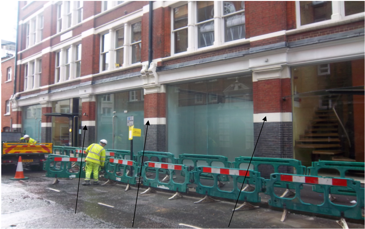
3. Close up of the shopfront and proposed position of the three wall lights
