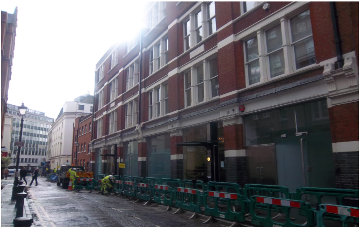
2. View of the existing shopfront
