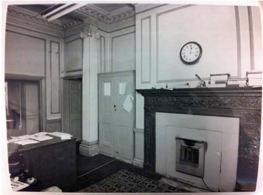
Figure 11: Ground floor room of no. 14 Southampton Place (1970)
