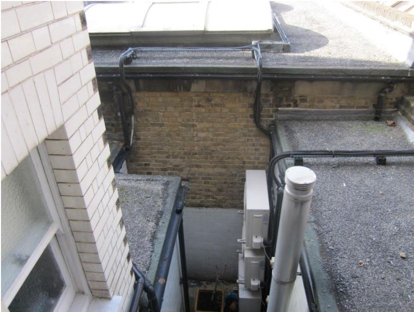
Figure 1 – Existing plant location at rear of 17 Doughty Street
