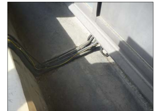
Survey photos of proposed location
