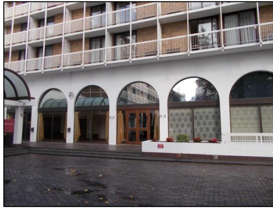
Location for proposed new ground floor brille soleil and decorative treatment to Pre-function entrance
