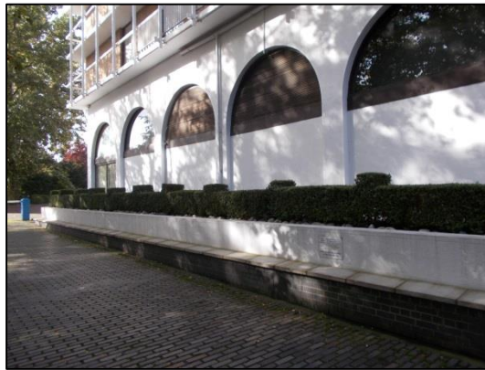
Location for new doors in Pre-function and Adelaide Suite
